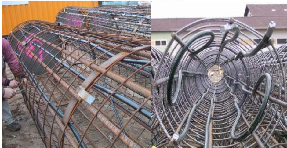
Figure 7: Sketch of an energy pile and view in a rebar cage for an energy pile (from http://www.spezialtiefbau.bilfingerberger.de [7])
