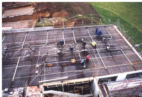
Figure 12: Pictures of vertical loops and concrete core activation (from VIKA [10])
