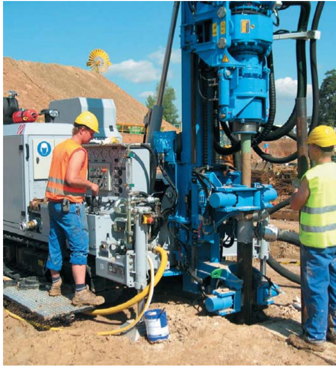
Figure 4: drilling for borehole heat exchanger (from: http://www.Prakla.de [4])
